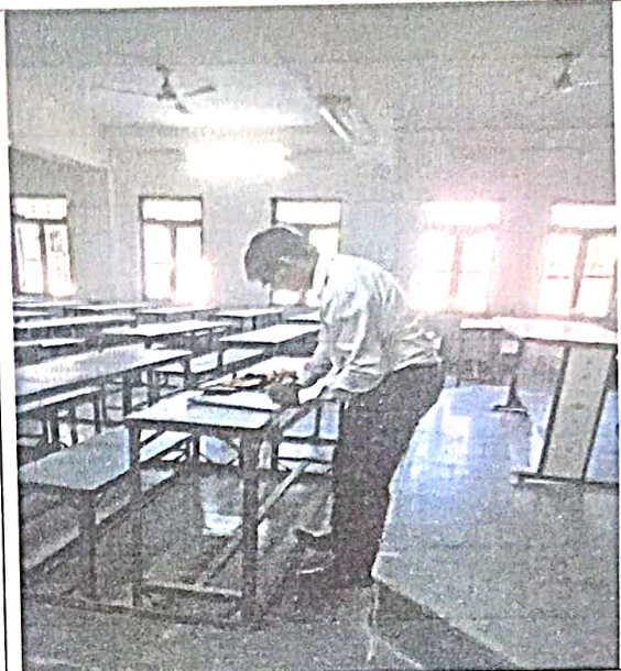
Proper Lighting Fitting & Connection for Fan
